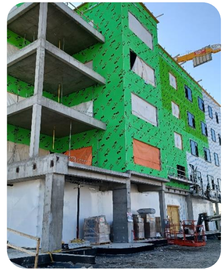
Northwest corner of building. Ready for vapour barrier and window install.
