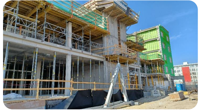
Front view of facility. Construction of concrete structure underway.
