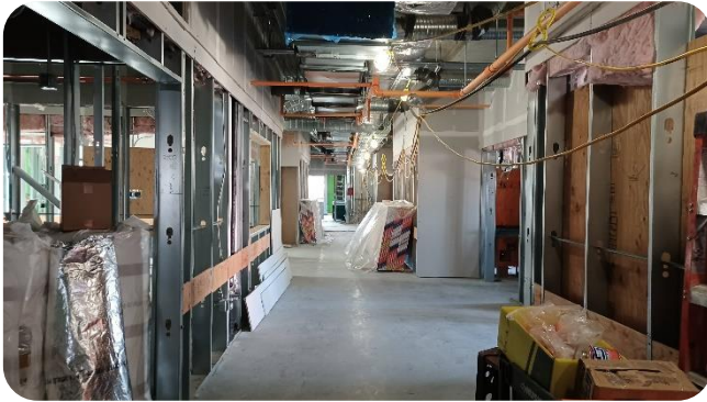
West Tower framing, rough-ins for plumbing, HVAC, and electrical underway.
