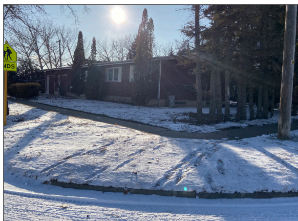
Figure 4: Example of a sidewalk that does not have curb ramps to allow all pedestrians to cross the street.
