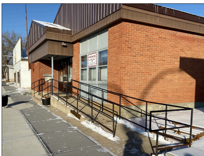
Figure 10: Example of an accessible building entrance.
